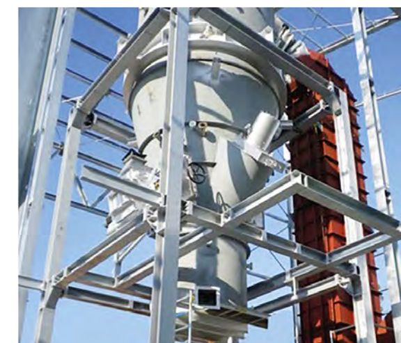
Thermal utilization of municipal sludge, City of Mainz (DEU)
