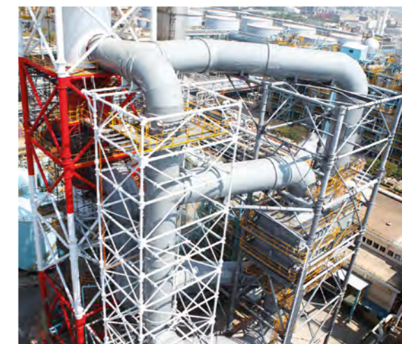
PFA coated heat exchanger for use in corrosive media, CPC (TWN)
